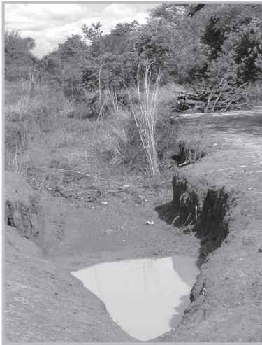
Gully resulting from erosion
