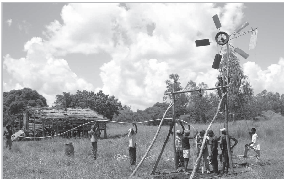
Wind rope pump being erected at Nhama-tanda in Mozambique
