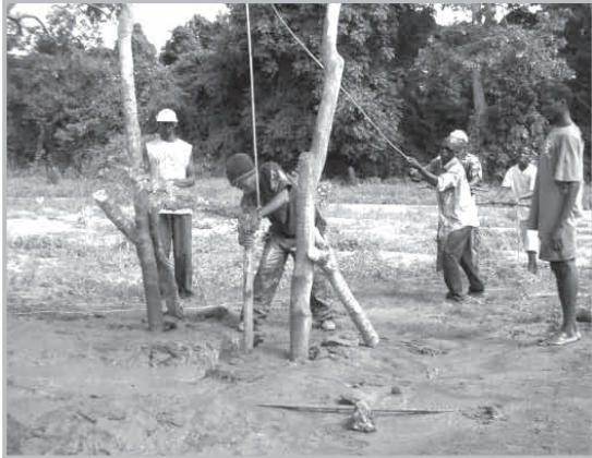
Drilling a borehole with the "Baptist" system in Mozambique
