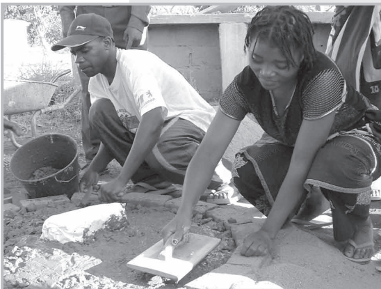
Producing a slab for a latrine of the kind in which a tree will later be planted
